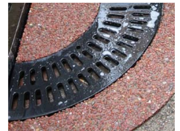
Even the gutters in front of the building are shaped to echo the arched roof.
